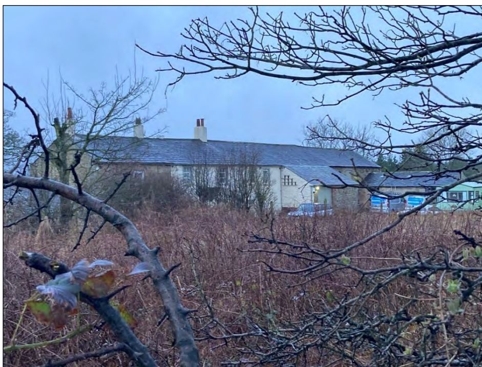
Figure 6.6: The northwest elevation of Wythemoor Sough (Grade II Listed)
